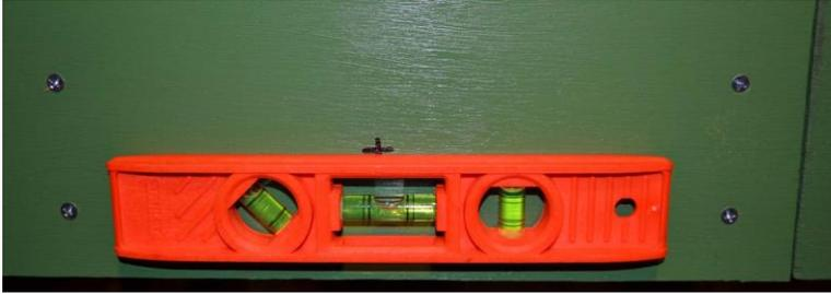
*Photo 2: The center point of the panel has been marked. Then, a small level was used to mark a horizontal line. After that, the two centers for the pilot holes were marked one inch apart.*
