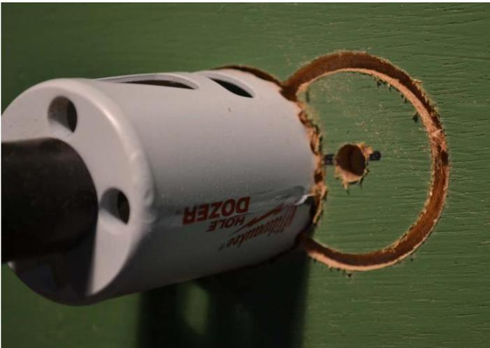
*Photo 4: Using the pilot holes as guides, the 1 ½” hole saw is used to drill the larger holes.*
