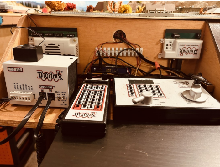
Photo 11: Command Control Station.
