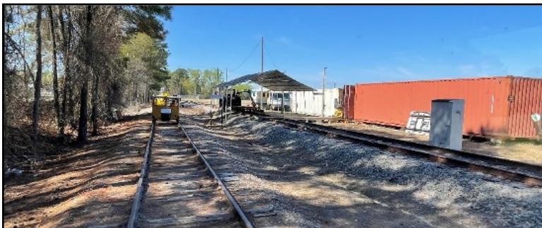
Photo 14: Hollis siding is a railcar storage facility. Members can trailer their speeders or garage them in a storage container.
