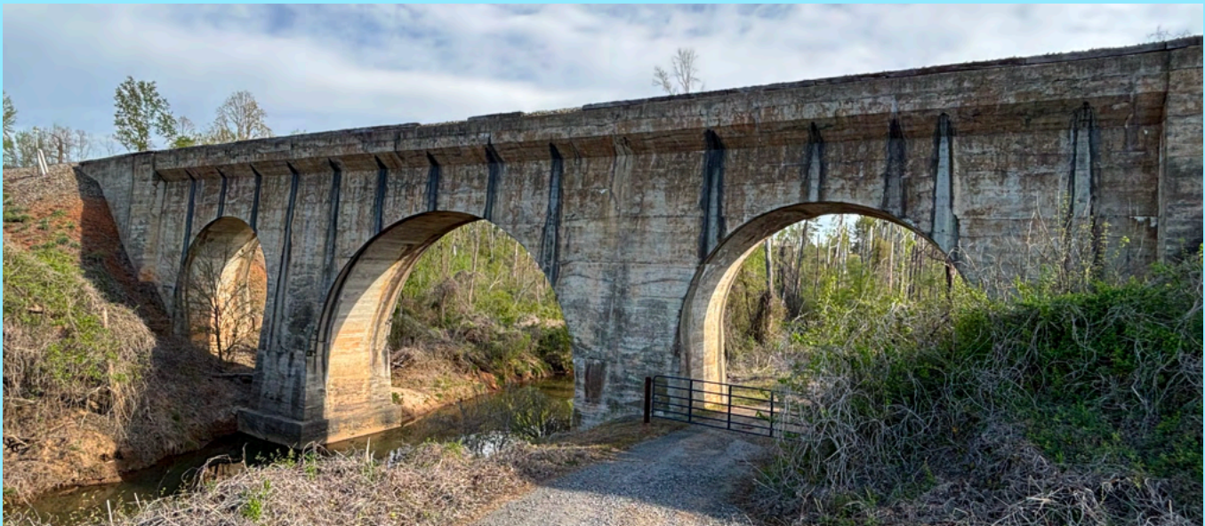
Photo 1: Streetside View of McLin Creek Viaduct
