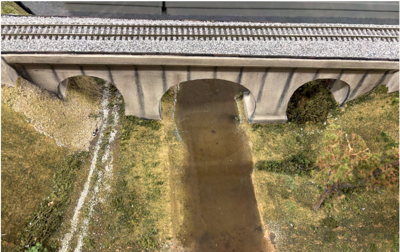
Photo 8: Overhead View of the Creek
